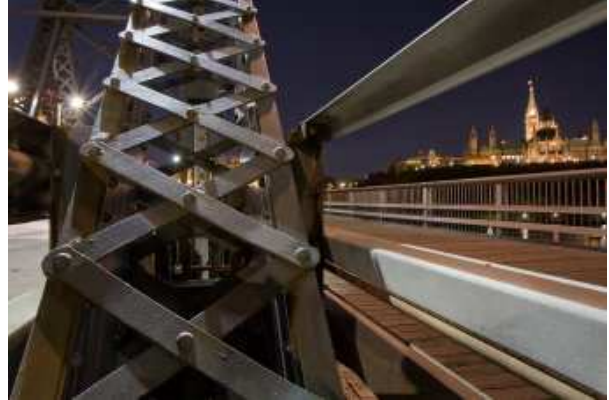
Alexandra Bridge Ironwork, Ottawa, Ontario
